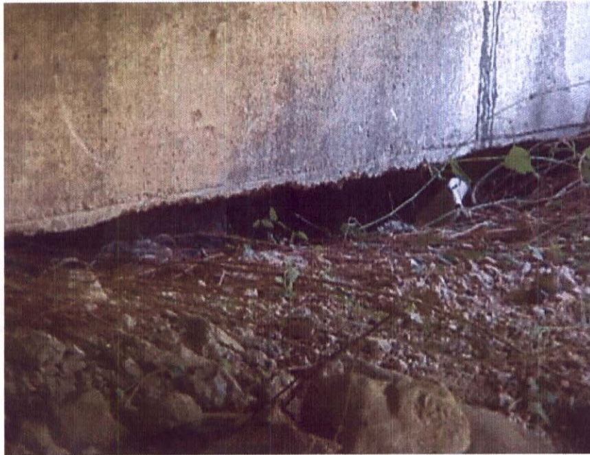
ABUTMENT #1 EMBANKMENT UNDER CAP
