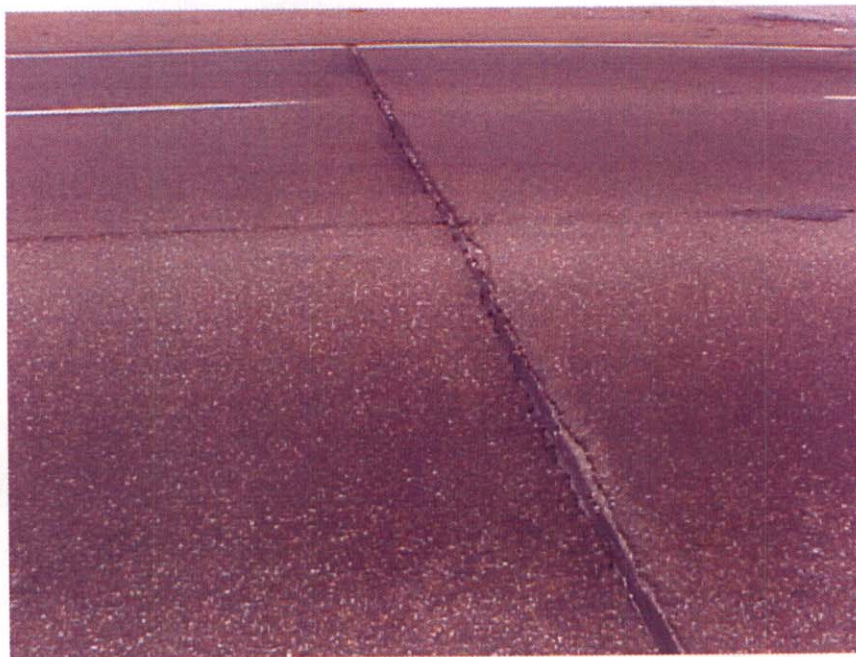
APPROACH #2 ASPHALT SPALLING AT JOINT
