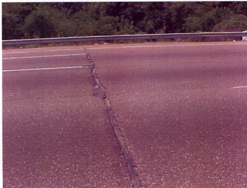
APPROACH #1, ASPHALT SPALLING AT JOINT
