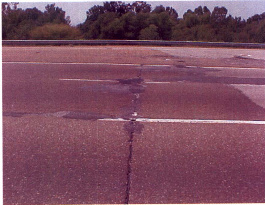
APPROACH #2 ASPHALT SPALLING
